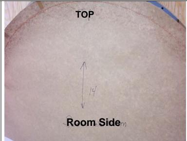
5. Cut the shape from the paper. Place the template back into the window opening to check for proper fit completely around.
